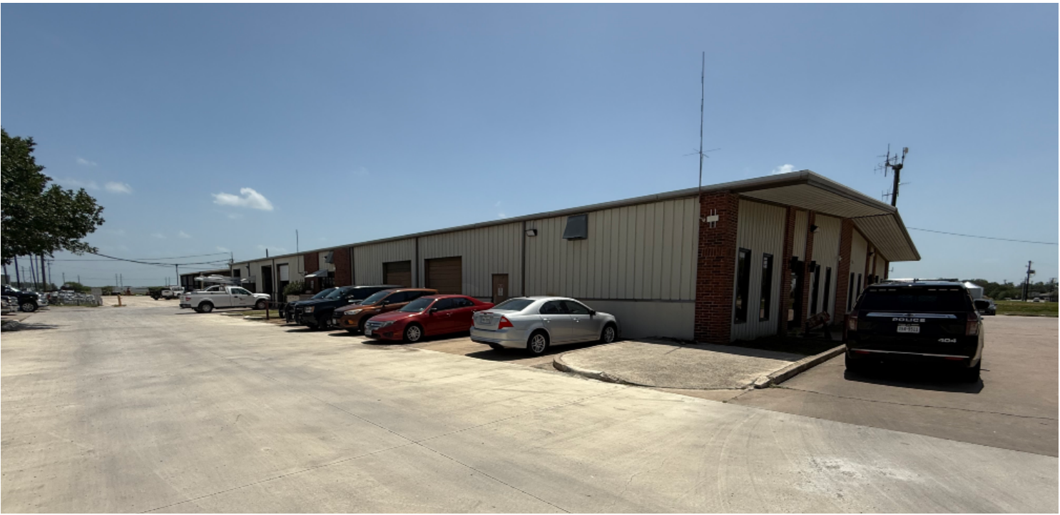
PHOTO OF EXISTING BUILDING
