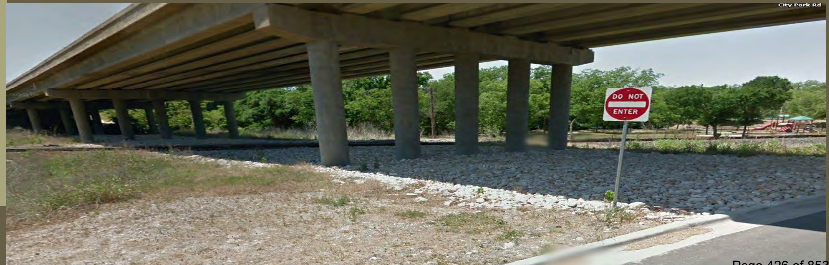
-US183 – Overpass over the Railroad
