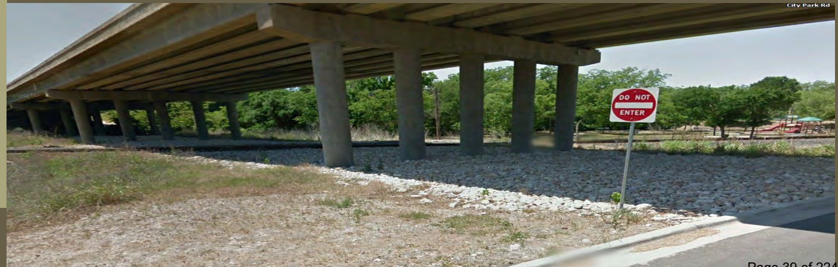
-US183 – Overpass over the Railroad
