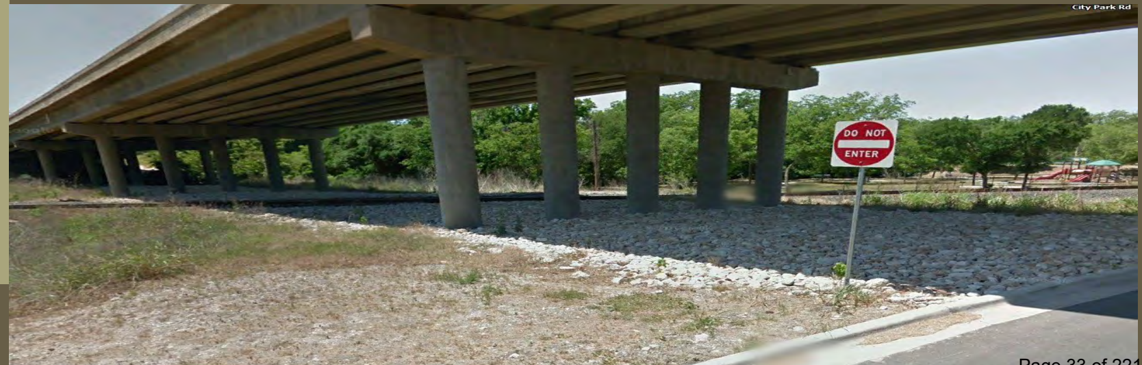
-US183 – Overpass over the Railroad
