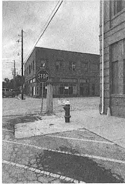
Existing fire hydrant location
