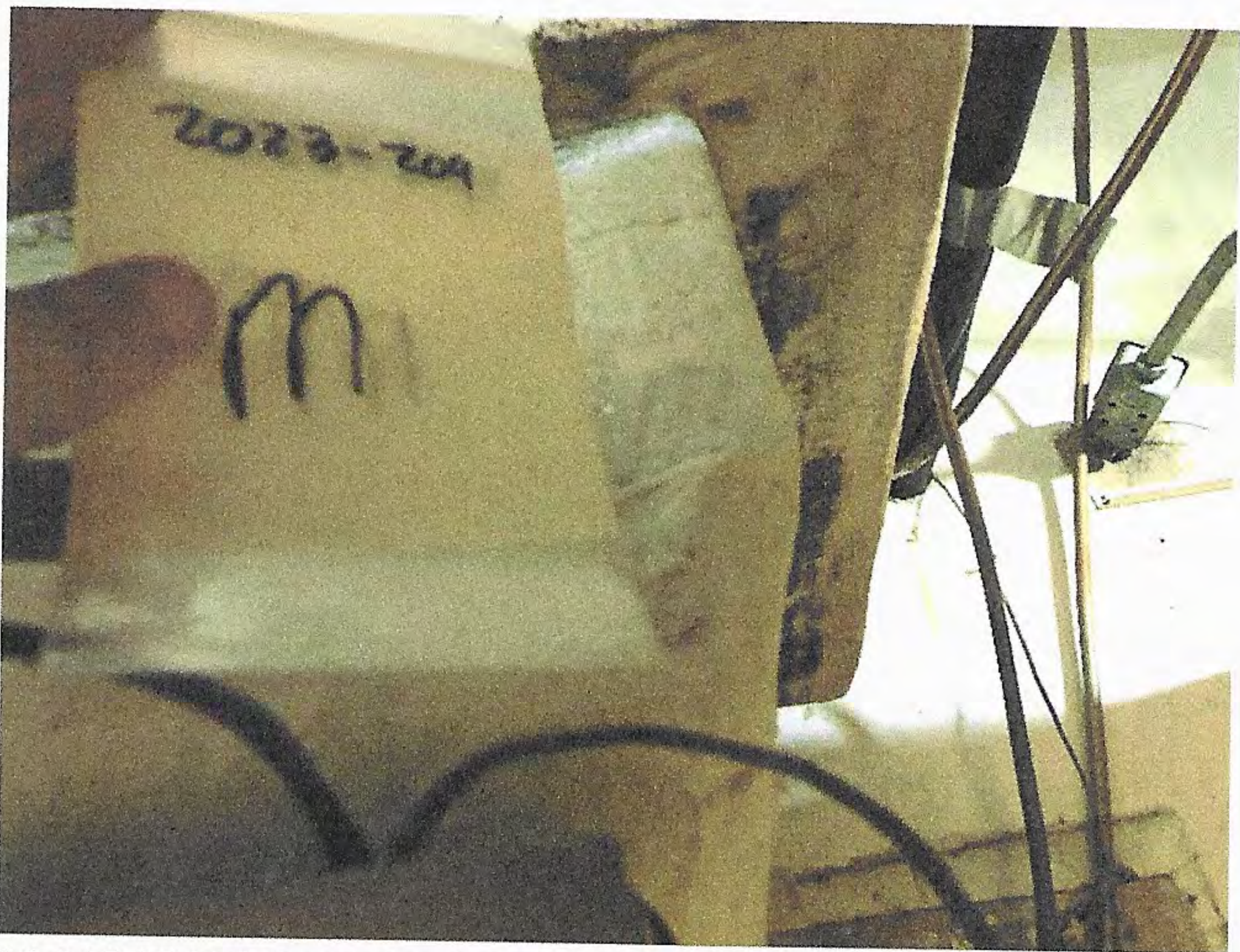
M-M2 HVAC Duct Sealant Mastic
