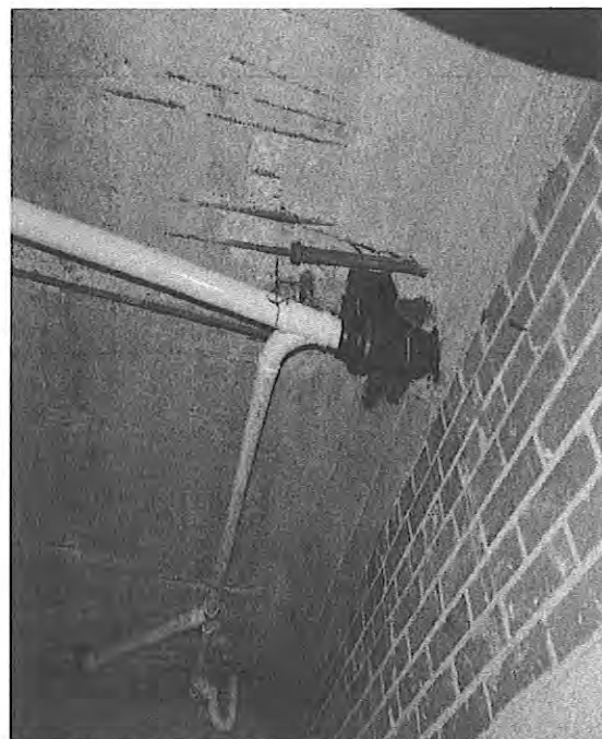
Sanitary piping under second floor
